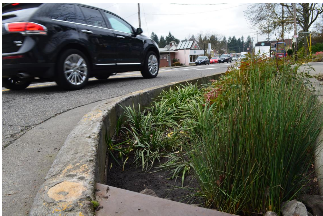
Figure 10.2 Bio-swales with low maintenance native vegetation improve roadside aesthetic while providing water storage and filtration services (Source: Barton, A.).
